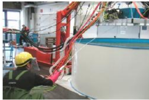
Shower watering during operation
